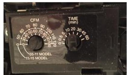
The CFM rate can be increased when indoor humidity is high or there are odors in the home. The fan's activation period can be made longer if the
